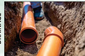
UNDER GROUND DRAINAGE
