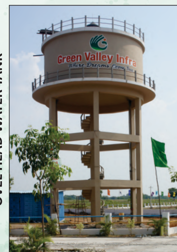
OVER HEAD WATER TANK
